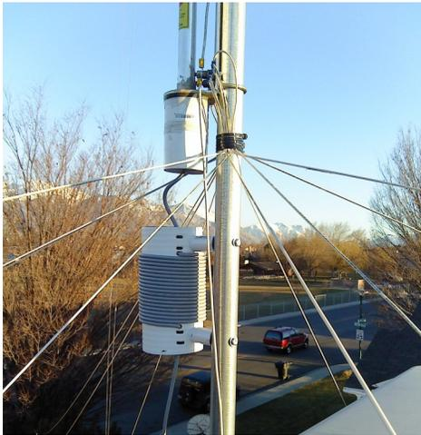
*The "Ugly Balun", installed under a vertical HF antenna*
