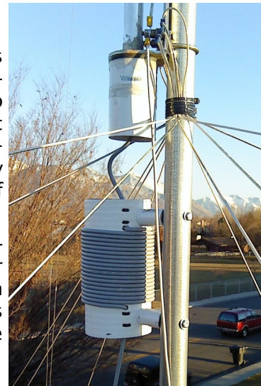
DIY current balun on my HF mast (wires are radials)
